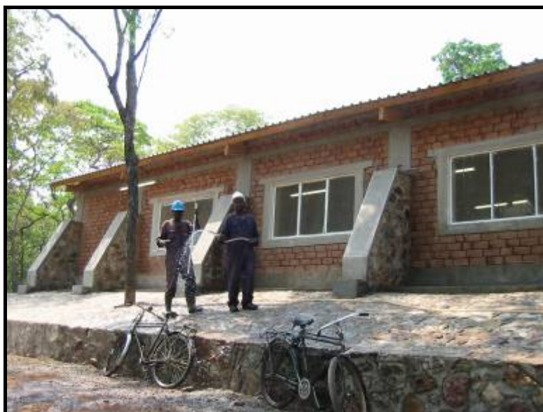
Completed mess building at Kinsevere mine site. (photo Oct 20, 2006)
