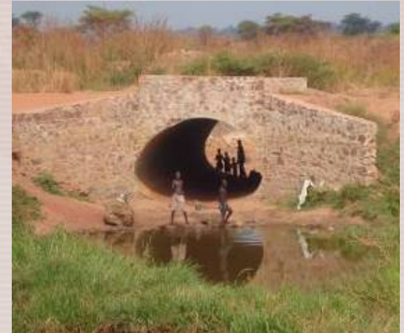
New Armco bridge
