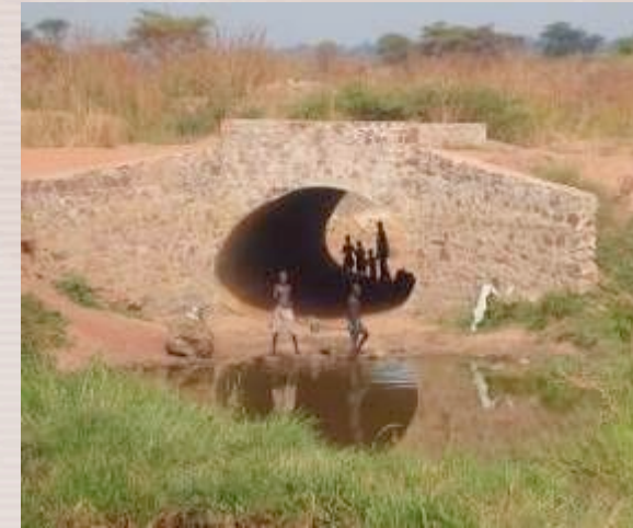
New Armco bridge
