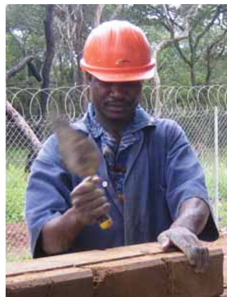
On-site brick making – Kinsevere
