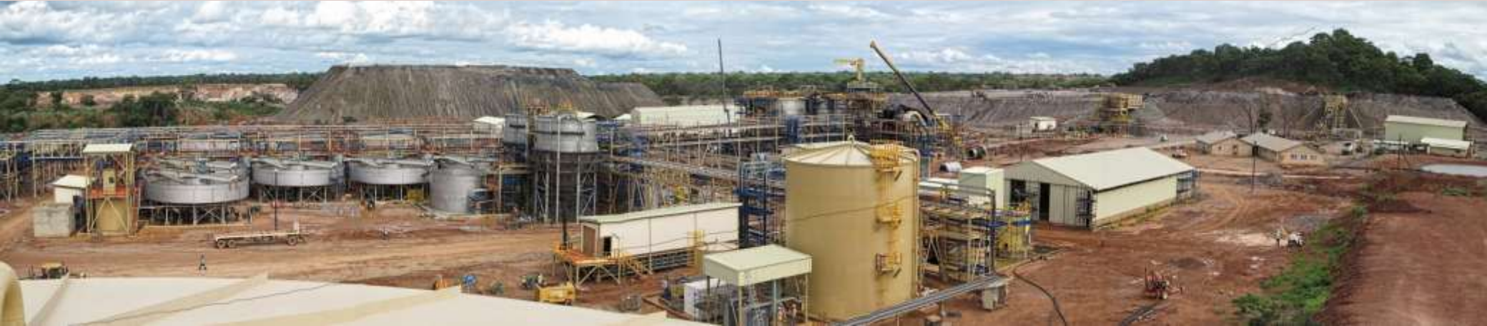
Kinsevere Stage II – Construction February 2011
