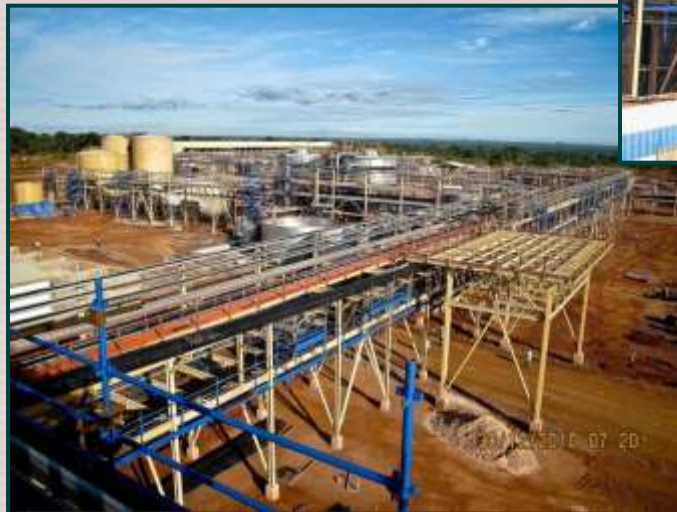
Main Control Room Structure
