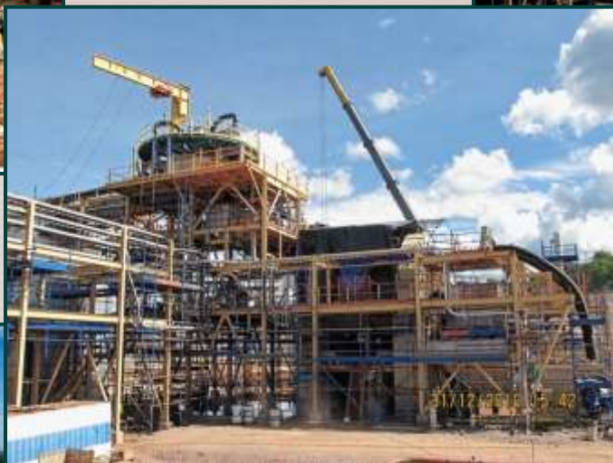
Mill & Cyclone Tower
