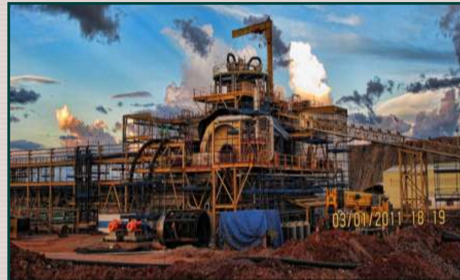
Mill & Cyclone Tower
