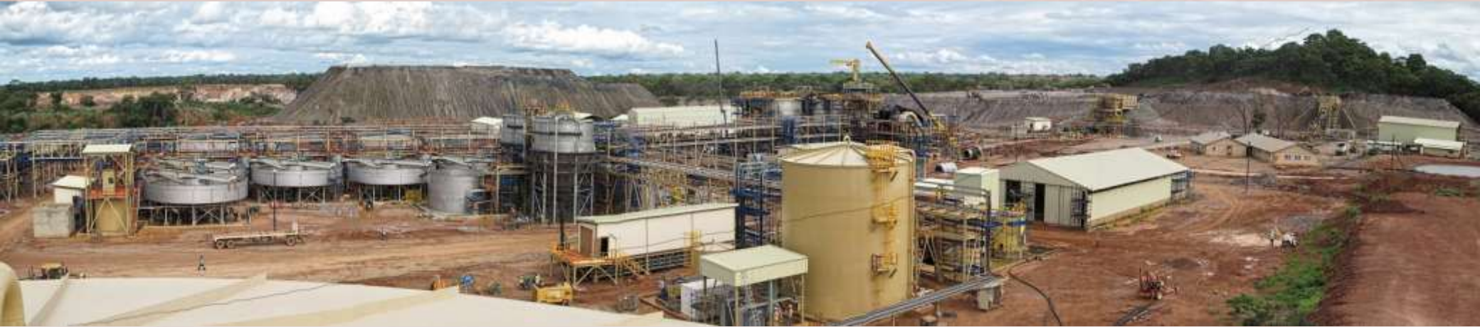
Kinsevere Stage II – Construction Q1 2011
