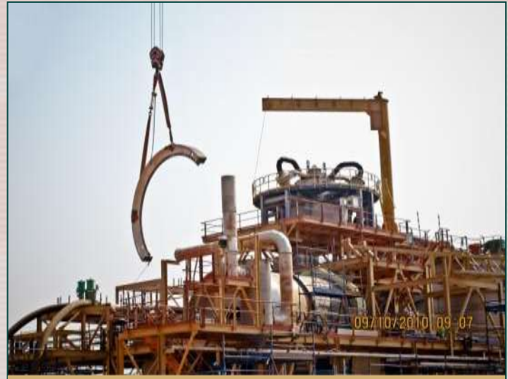
AREA 15 GRINDING - INSTALLATION OF RING GEAR
