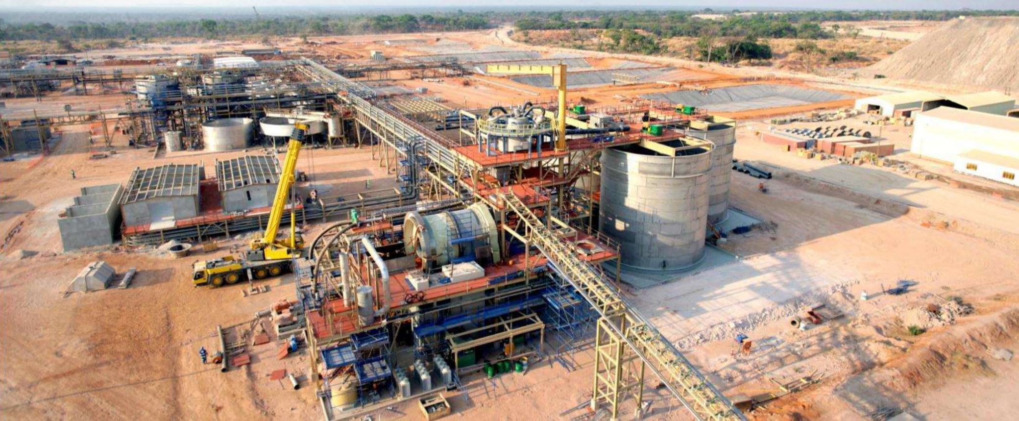
Kinsevere Stage II, 60,000 SX-EW in construction – Q3 2010
